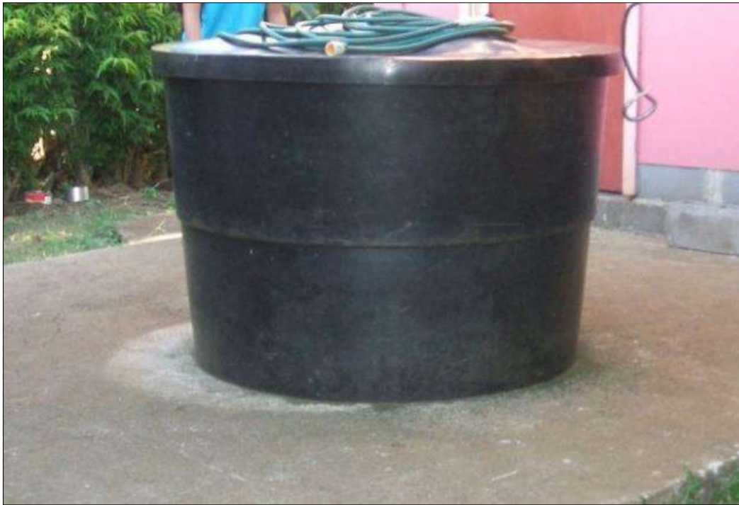
Figure 6.4: A family- owned water tank at Maagiagi.
