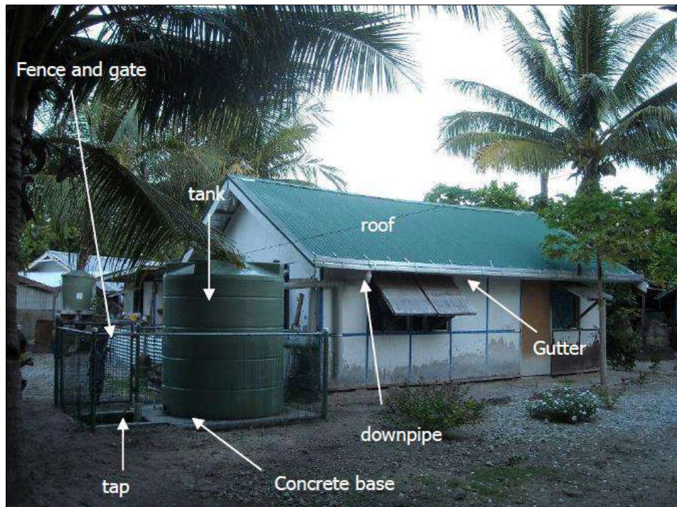
Figure 2.3: Different parts of an I-Kiribati household water harvesting system (GWP Consultants Limited, 2011).
