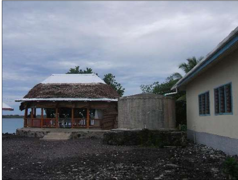
Figure 5.8: Cement water tanks built after the 1990s cyclones.
