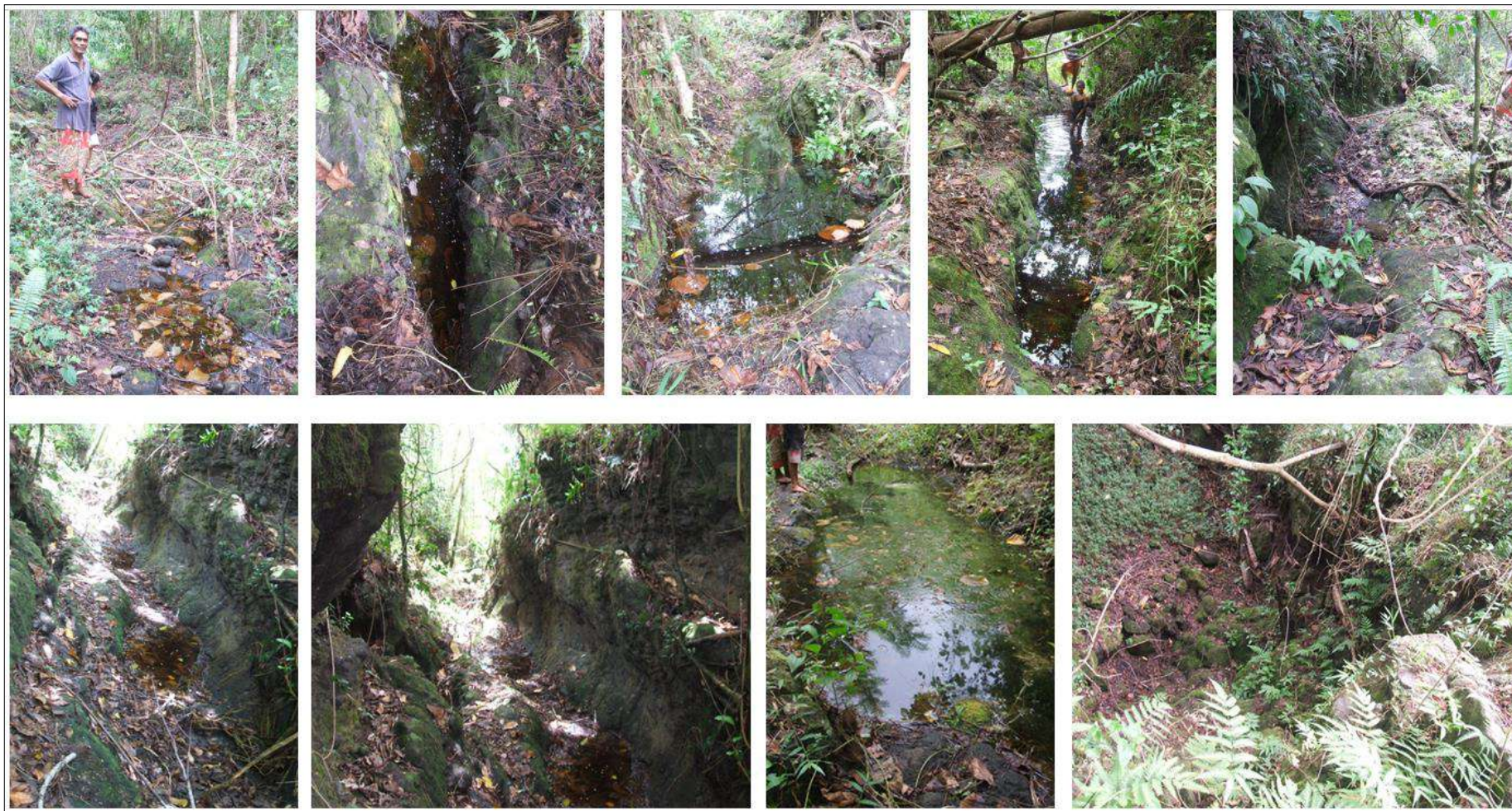
Figure 6.11: A local chief indicates that many more parts of the Aopo stream had dried up during the dry seasons of recent years.
